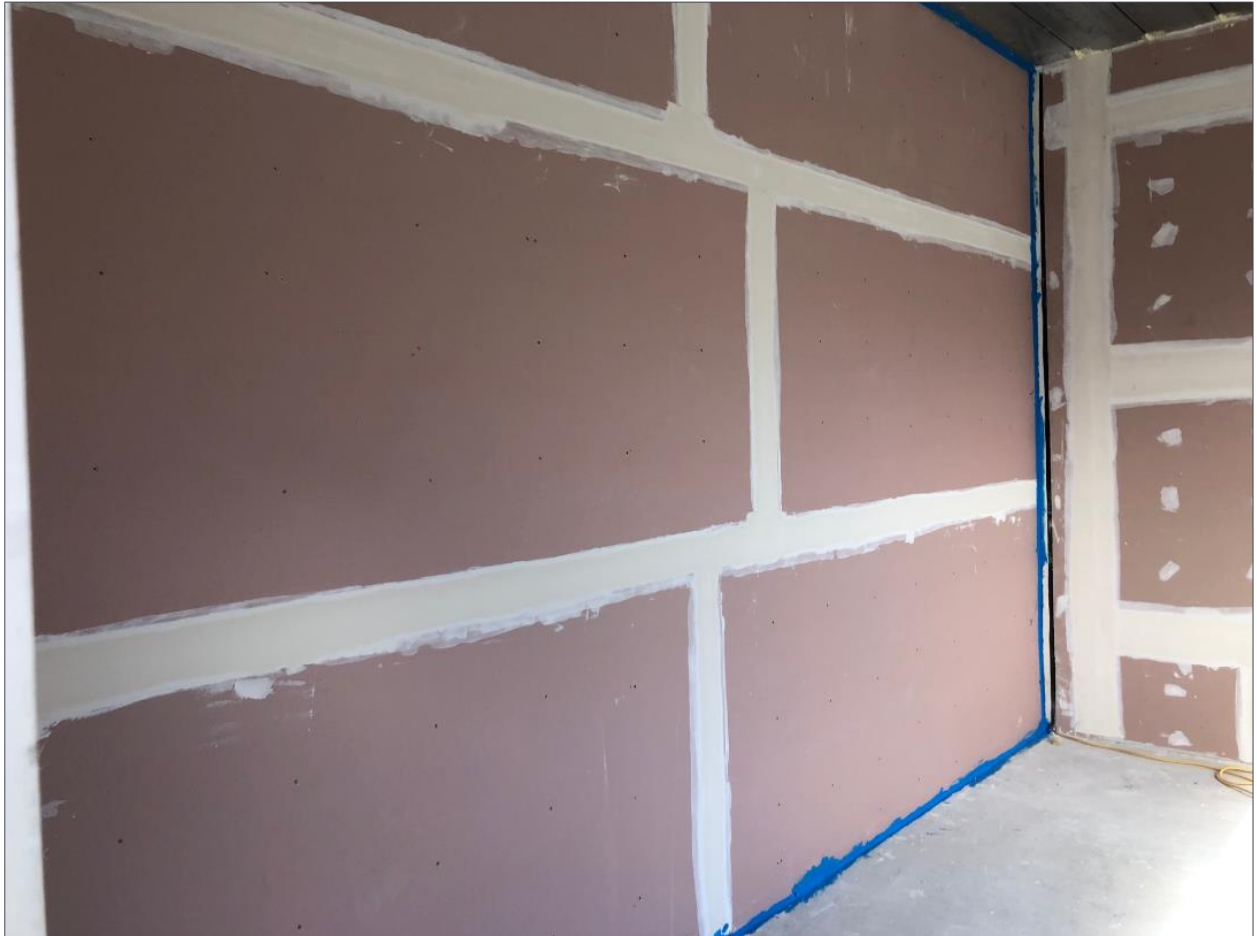
Figure 4: Source room side of wall
