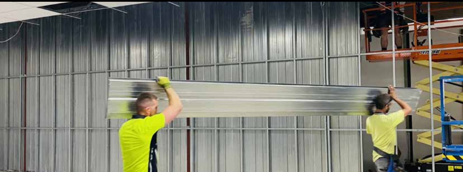
K8 SUPAPANEL® onsite install
